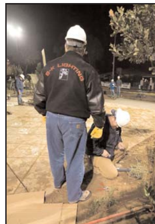
B-K Lighting President Doug Hagen supervises installation of outdoor lighting fixtures.
